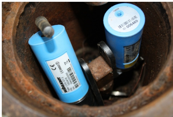
Log N-3 noise logger with magnetic angled adapter and GSM transmitter with magnetic angled adapter and 90-degree antenna adapter in a German gate shaft.
